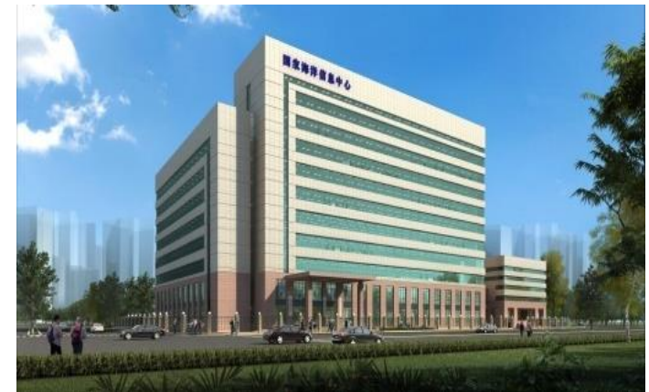
New Look after Energy-saving Reconstruction since September 2016
